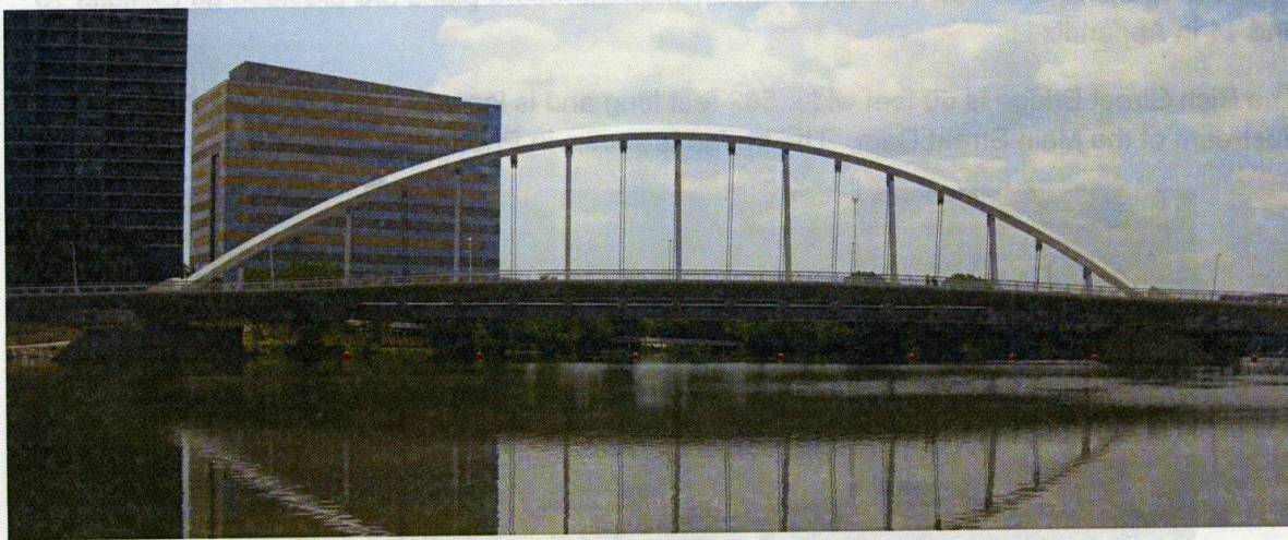
Photo 8-2. Main Street Bridge (looking south)
