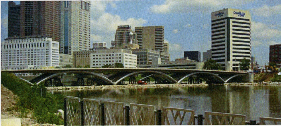
Photo 8-3. Rich Street Bridge looking north
