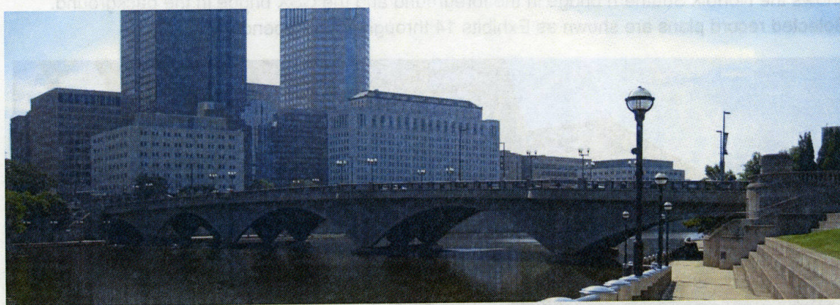
Photo 8-4. Broad Street Bridge looking south
