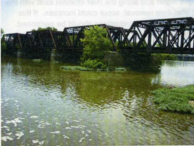
Photo 8-1. NS/CSX Bridge showing aggradation at pier
