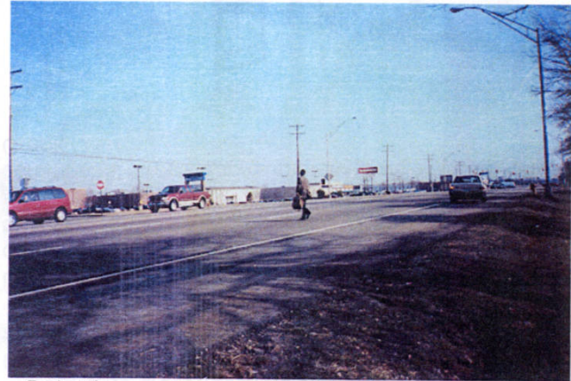
Pedestrian crossing Morse Road in front of Northland Mall.
