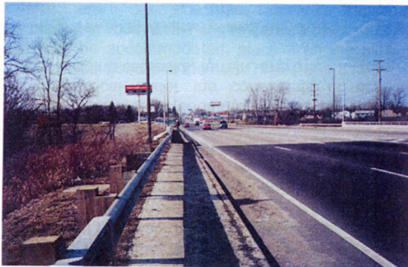
Morse Road bridge near Sunbury Road
