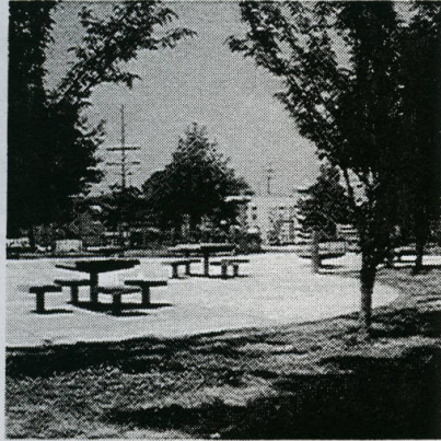
Weinland Park is the largest active park in the Neighborhoods.
