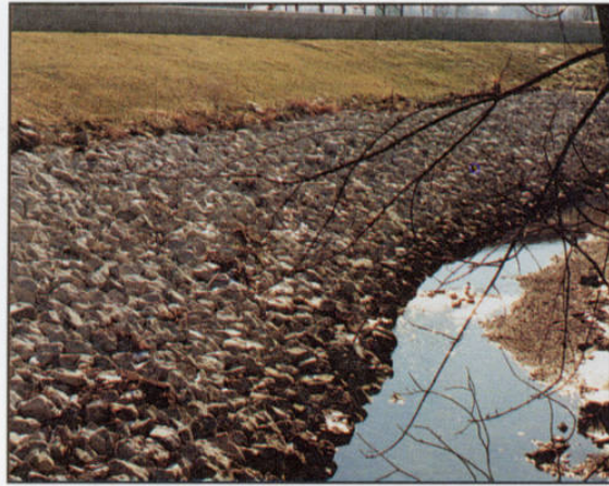
(Fig. 34) Flood wall at Dry Run
