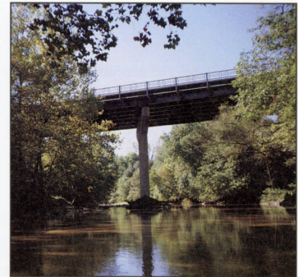
(Fig. 62) Bridge crossing high above Alum Creek
