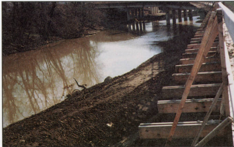
(Fig. 17) Construction sites can be major sources of erosion and sedimentation
