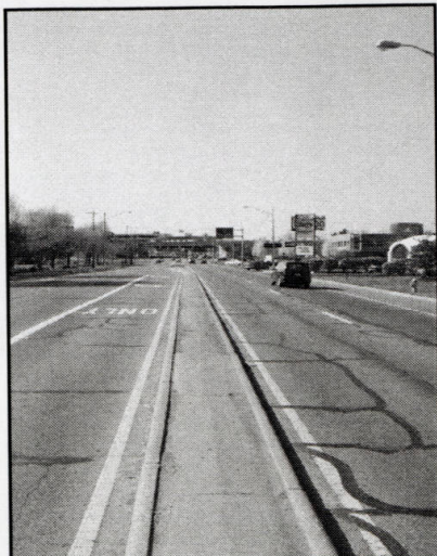
Existing concrete median.
