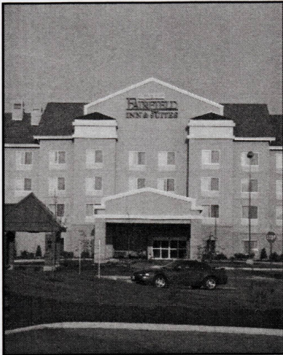
The new Fairfield Inn was constructed on the site of a former hotel. The Inn exemplifies the continued viability of hotels in the Olentangy River Road corridor.
