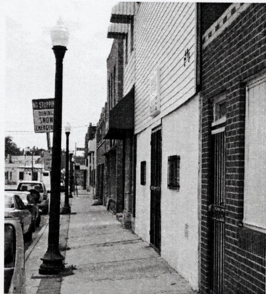
Existing commercial structures on Cleveland Avenue.
