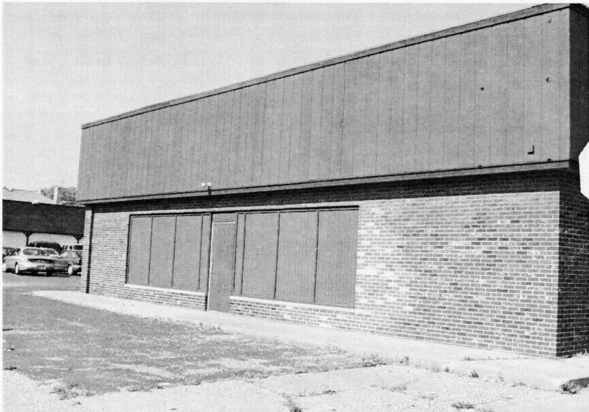
Example of a vacant commercial building on Cleveland Ave.
