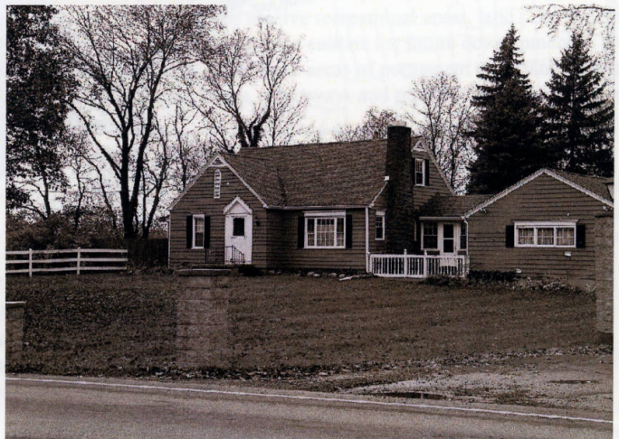
Residential building on Brown Road
