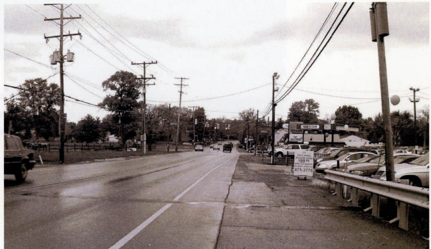
Many area roads lack sidewalks
