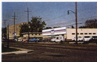
View Northeast to Post Office
