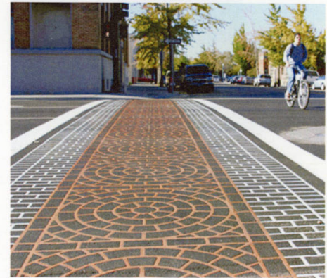
Example of textured cross walk pavement.
