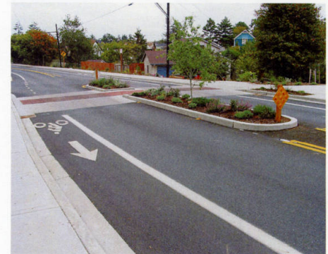
Example of "Road Diet" that incorporates bike lanes and a planted median.
