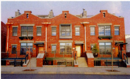
Example of multifamily housing that contributes to street life through the use of front stoops, and other means.
