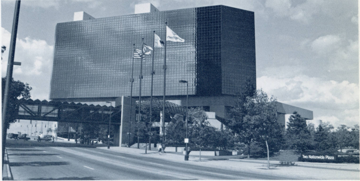
The Ohio Center and the adjoining Hyatt Hotel, major activity centers at the northern end of High Street.
