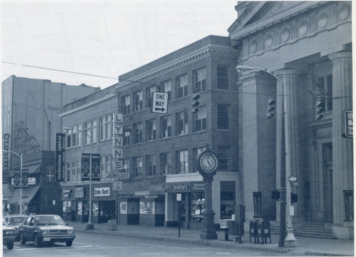
Retail establishments along High Street in downtown Columbus.
