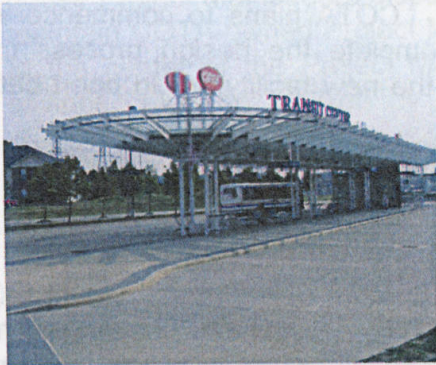
Easton Transit Center
