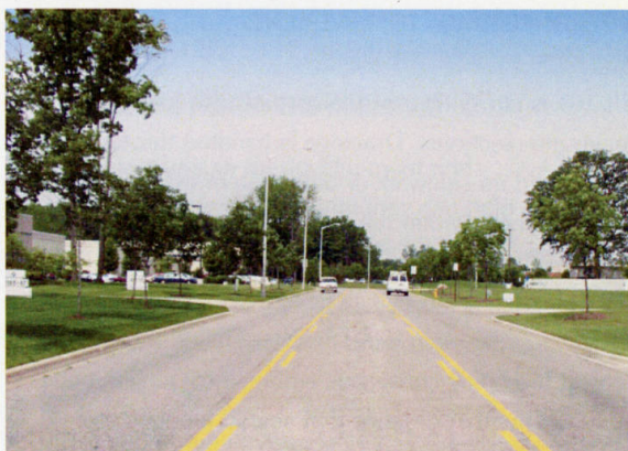
Three-lane road Two moving lanes of traffic with one center turn lane.
