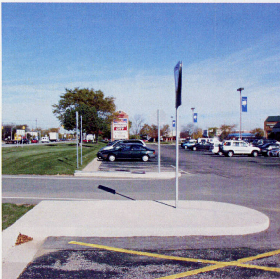
Commercial area with no sidewalk access.
