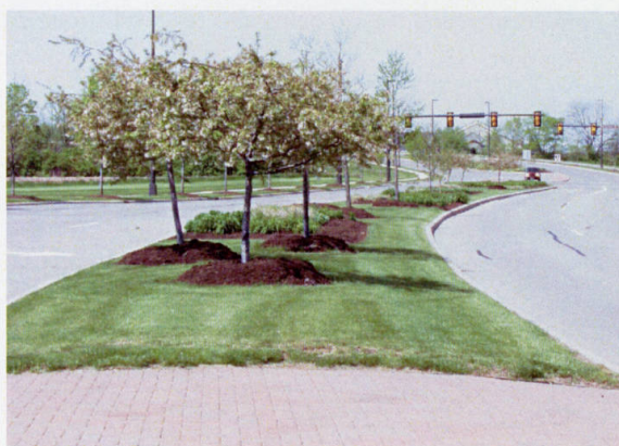
Five-lane road with landscaped median Two moving lanes of traffic in each direction with one center turn lane. Landscaped median located where the turn lane is not necessary.
