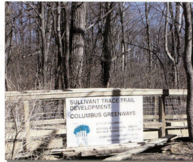
Construction of Sullivant Trace Trail
