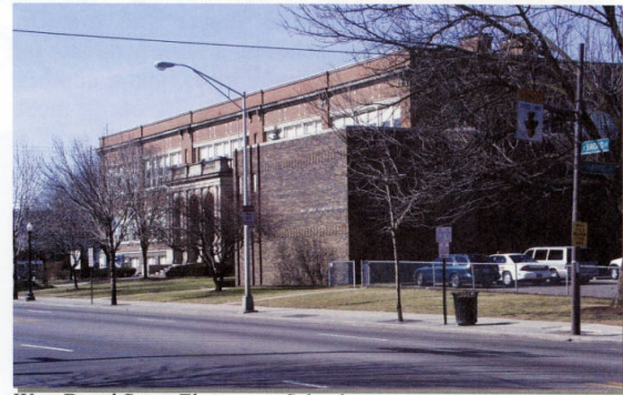
West Broad Street Elementary School
