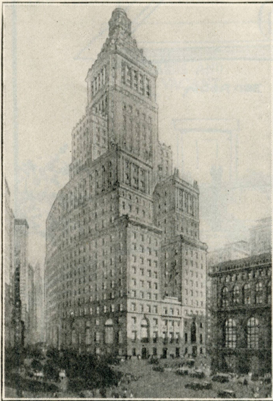
Standard Oil Building, New York City, Showing how a Zoning Ordinance Insures Light and Air to Surrounding Buildings as well as to the Building Itself
